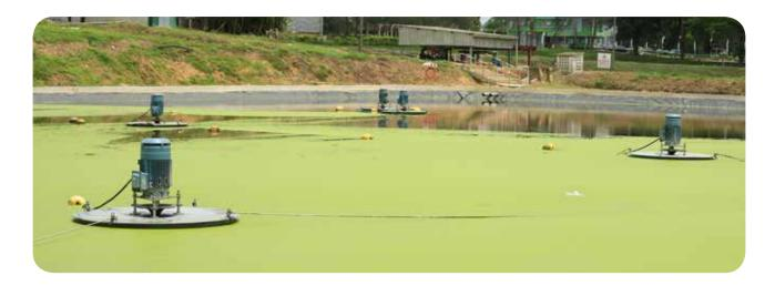
For many years, SIPH has been striving to reduce water consumption for an equivalent volume of activity by implementing recycling into the industrial process. Thus, methods of recycling used at most SIPH Group factories include reusing the process water from the last basins for prewashing cup bottoms. The reduction in water consumption 2020-2021 is -8%.
